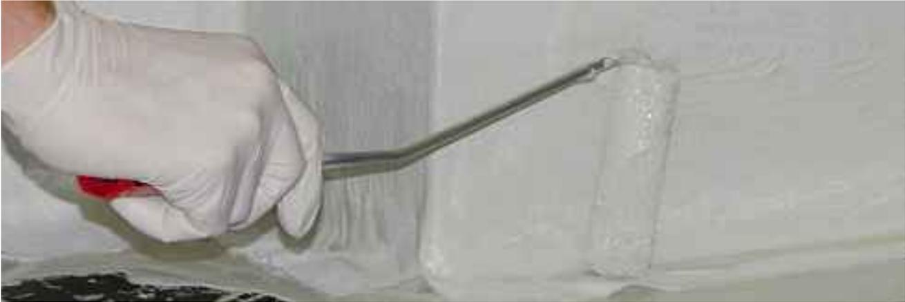
Liquid applied **Sikalastic**® membranes can be used in conjunction with glass reinforcement mats, to provide seamless waterproofing around all different types of detailing at areas including: upstands, plant and equipment entries, or around other roof penetrations and components.
