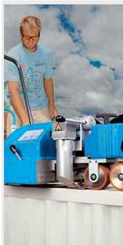
Automatic welding equipment is used to weld membrane seams safely and efficiently, with high quality and reliability, particularly on large flat areas. The welding and equipment parameters always need to be adapted to the site conditions. The welding machines developed for use with Sika membranes allow adjustment to suit almost any weather conditions, including high humidity or for welding in the wet and in very cold weather, even at temperatures below 0 °C.
