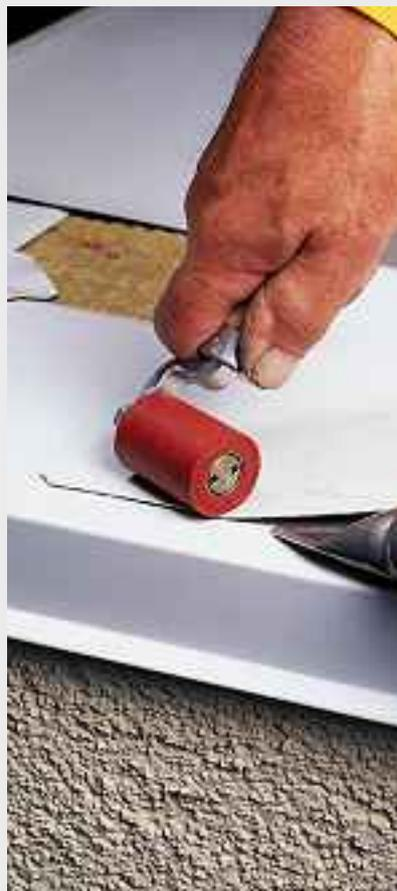
Laminated metal sheets consist of galvanized sheet metal laminated on the top side with **Sikaplan®** or **Sarnafil®** membrane. The lamination has the same properties and compatibility as the roofing membrane sheets. The laminated metal sheets can therefore easily be welded to the waterproofing membranes during installation.
