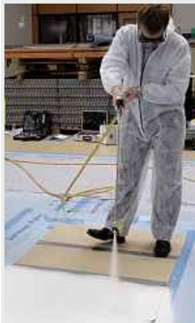
In addition to roller application the 1-C PU liquid applied membranes can also be applied with airless spray equipment. This method is used for the **SikaRoof® MTC 8** System and top coat applications in other **SikaRoof® MTC** Systems. Two spray applied coats are still the minimum requirement to ensure the correct thickness is applied.
