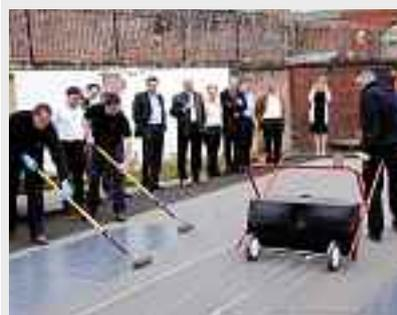
To speed up the application of 1-C PU liquid membrane applications on large areas, a special tool – the **Sikalastic® Applicator** has been developed. By using this innovative Sika equipment, roofing contractors can significantly increase their rate of application and reduce costs on large open roof spaces.
