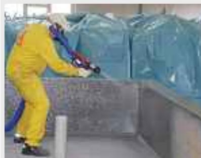
2-C PU liquid applied membranes are usually machine applied through hot spray equipment.
