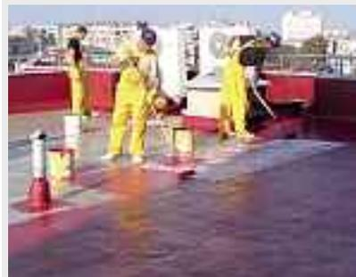
1-C PU liquid roofing membranes are mainly applied by roller and brush (brushes are always used for detailing).
