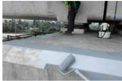
Bridge project in Malaysia
