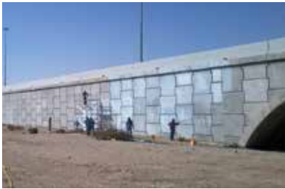
Bridge project in Qatar
