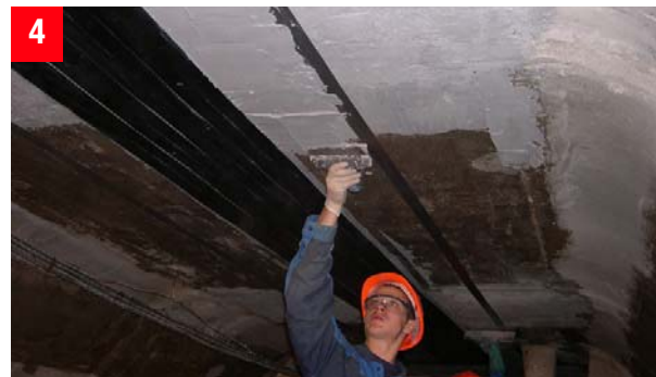
4 Sikadur®-30 epoxy adhesive applied to the substrate
