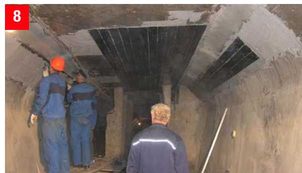
8 Finished application of the first 15 Sika® CarboDur® CFRP Plates Type S1214
