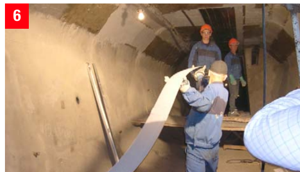
6 Taking a Sika® CarboDur® plate to its position
