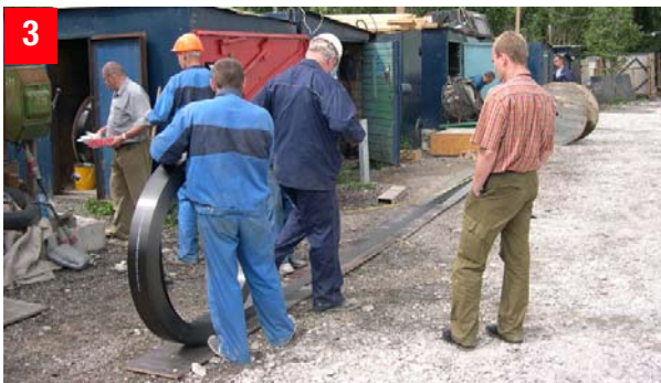
3 Preparing the Sika® CarboDur® CFRP Plates on site
