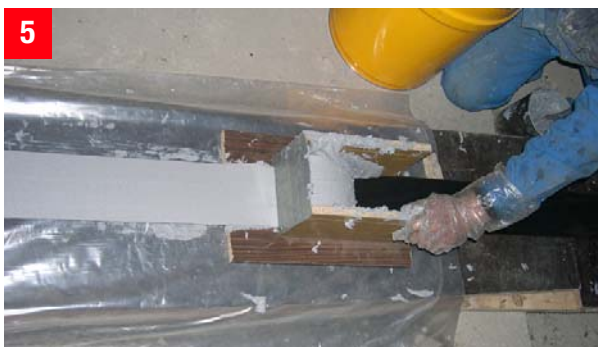
5 Coating the plate with Sikadur®-30 epoxy adhesive in a dome shape
