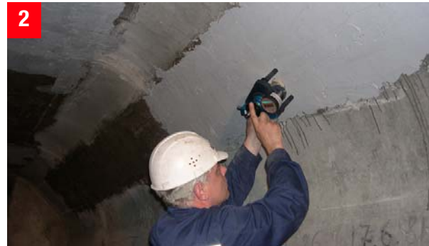
2 Pull-off test with steel dollies Ø 50mm
