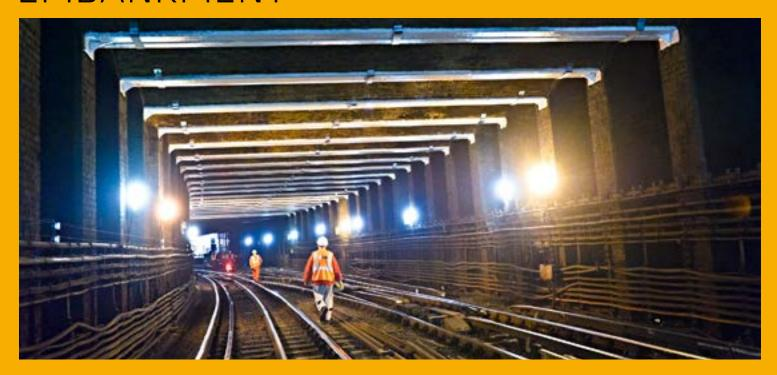
To minimise service disruption on the District and Circle lines, the entire process had to be completed during Engineering Hours (overnight when there is no train service) and was scheduled to be delivered in a series of shifts between 1am and 5am, over a period of six months. In each shift, the project team had to erect
