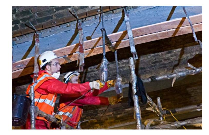
Specialist contractor, Contrete Repairs Limited carried out the skilled application, having been appointed by LU Framework Contractor, Clancy Docwra. The process began with each beam, measuring 7.5m long and 0.5m wide, cleaned using a powerful grit blasting technique that removed grease, oil, rust and any other contaminants which could reduce adhesion. Once dried, a coat of SikaCor®-EG 1 primer was applied, followed by the application of a resin to prepare the surface.
